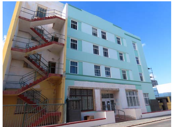
Main building renovations
